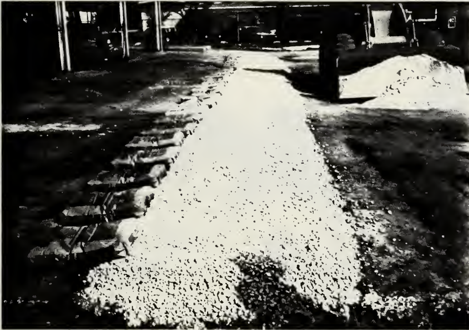
Figure 2.7 Cement Bag Placement
